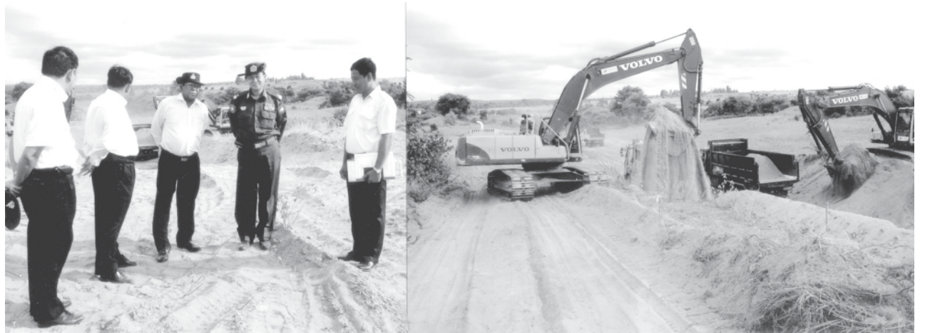
Minister Maj-Gen Aung Min inspects construction of Seikphyu-Pakokku railroad section.
