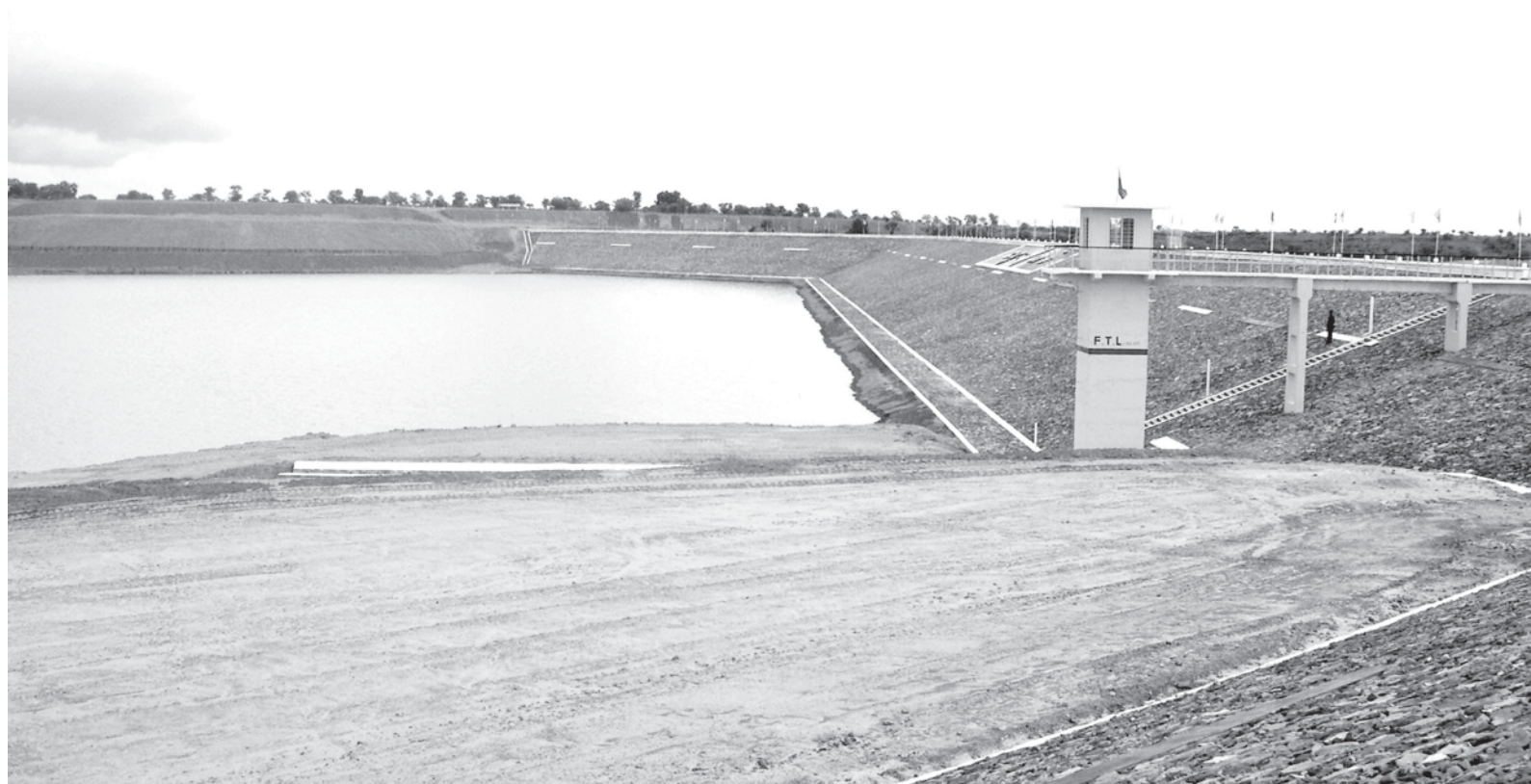
Gwaygyo Dam in Yesagyoo Township, Pakokku District. — A & I
