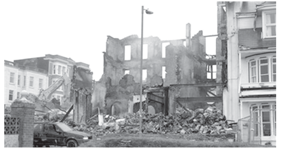
The partly demolished Penhallow Hotel in Newquay, Cornwall, England following a fire which broke out shortly after midnight on 18 Aug, 2007. Fire gutted a hotel on England's south coast on Saturday, and a man died after falling from an upper floor window, while at least four other people were missing, authorities said. Two hotel guests were being treated for critical injuries at a hospital, and at least four people were missing, police said. — INTERNET
