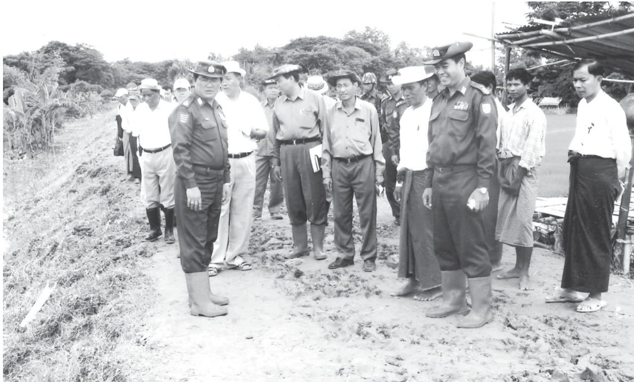
Commander Maj-Gen Thura Myint Aung inspects maintenance of embankments in Hinthada Township. — MNA
