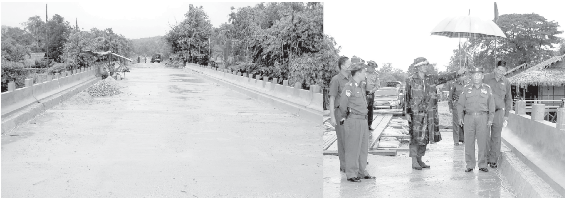
Lt-Gen Maung Bo inspects progress in construction of Yepone Bridge in Yebyu Township. — MNA
