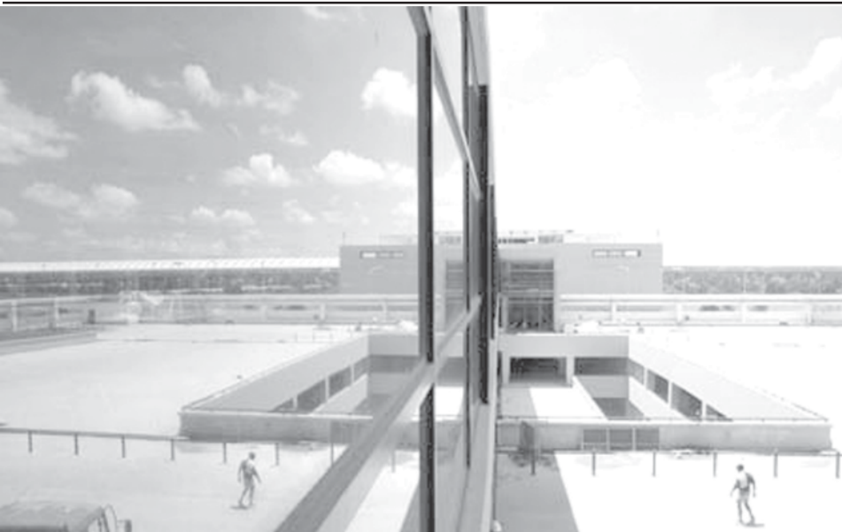
Photo taken on 7 Aug, 2007 shows the new decorated Terminal No 2 of the Pudong Airport in Shanghai, east China. As part of the expansion project of the Pudong Airport, Terminal No 2 has finished its fitment, entering the last stage of adjustment.—XINHUA
