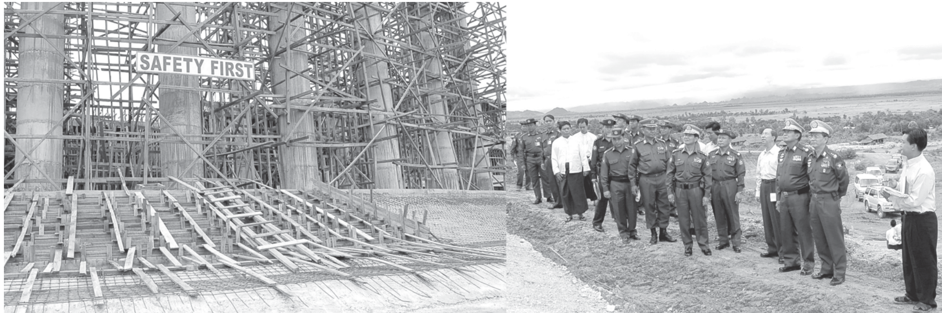
Secretary-1 Lt-Gen Thein Sein inspects construction task of Loikaw Technological University in Loikaw. — MNA
