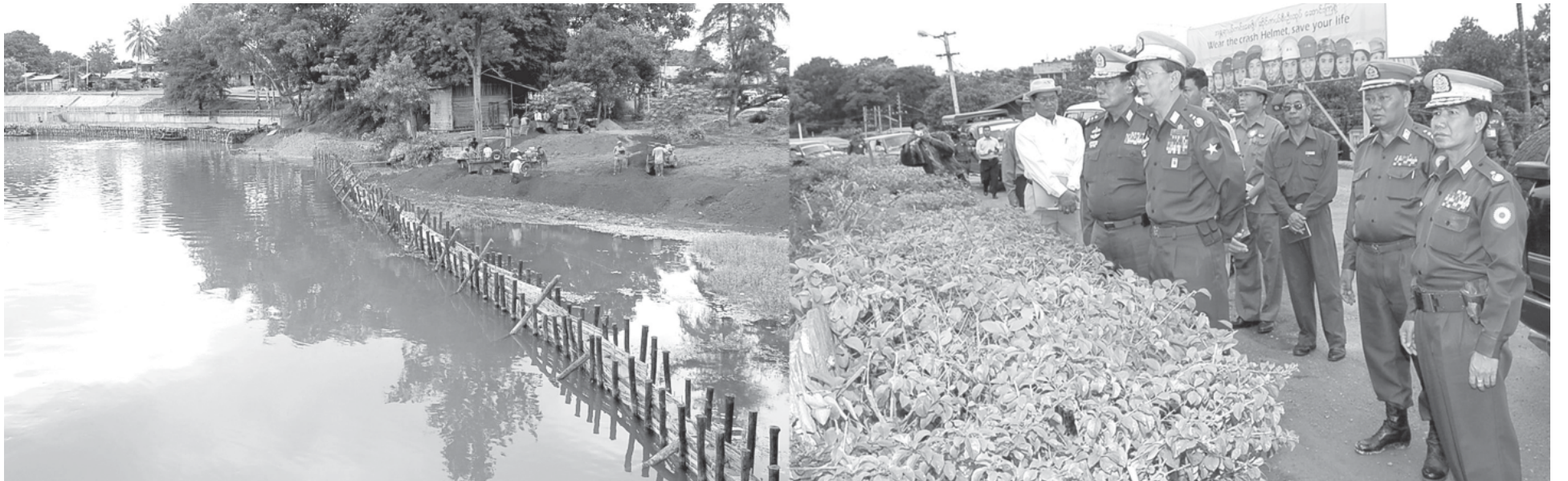
Secretary-1 Lt-Gen Thein Sein inspects construction task of retaining wall of Bilu Creek.— MNA
