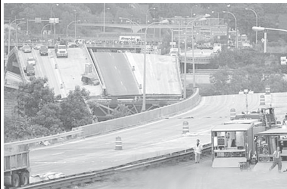
A freeway bridge over the Mississippi River in Minneapolis, Minnesota, collapsed on Wednesday, killing at least five people and plunging cars and tons of concrete into the water below. — XINHUA
