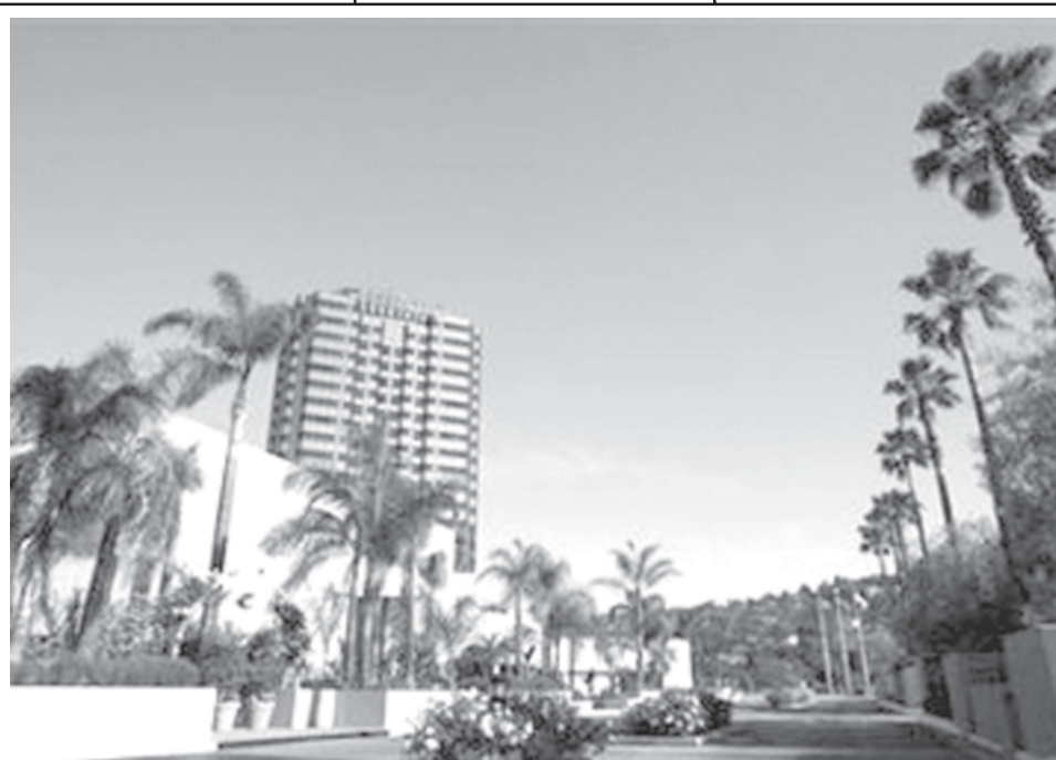
A general view of the Hilton hotel in the Universal City area of Los Angeles on 3 Aug, 2007. Buyout firms like Blackstone Group, which recently said it would buy Hilton Hotels, will have to adjust for less debt and will likely seek smaller deals. — INTERNET
