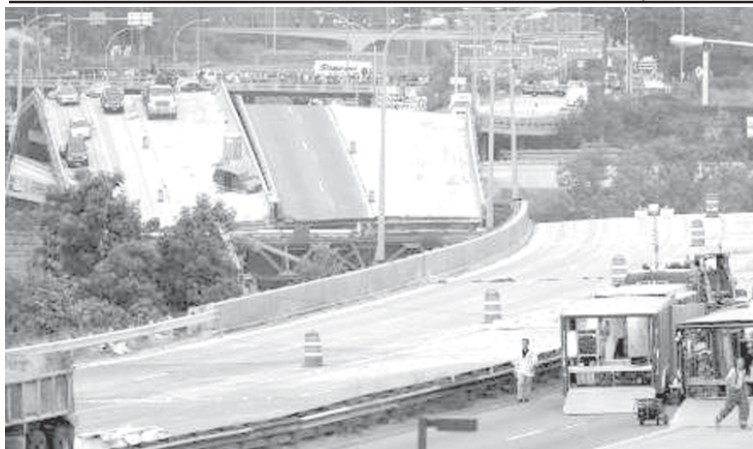
The I-35W bridge that spans the Mississippi River in Minneapolis, Minnesota, lies in pieces after it collapsed on 1 August, 2007. The highway bridge collapsed and hurled vehicles into the Mississippi River in central Minneapolis during evening rush hour on Wednesday, killing nine people and injuring dozens, officials said.—INTERNET
