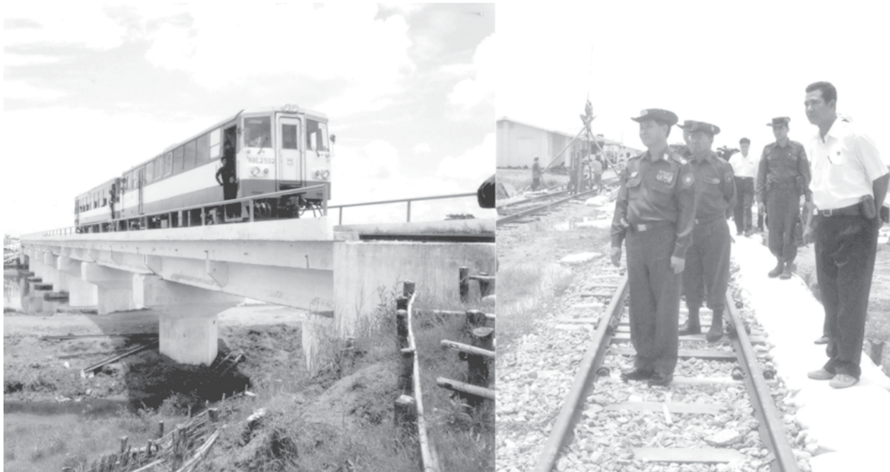
Minister Maj-Gen Aung Min inspects running a train on a bridge across Sittoung Tunnel. — MNA
