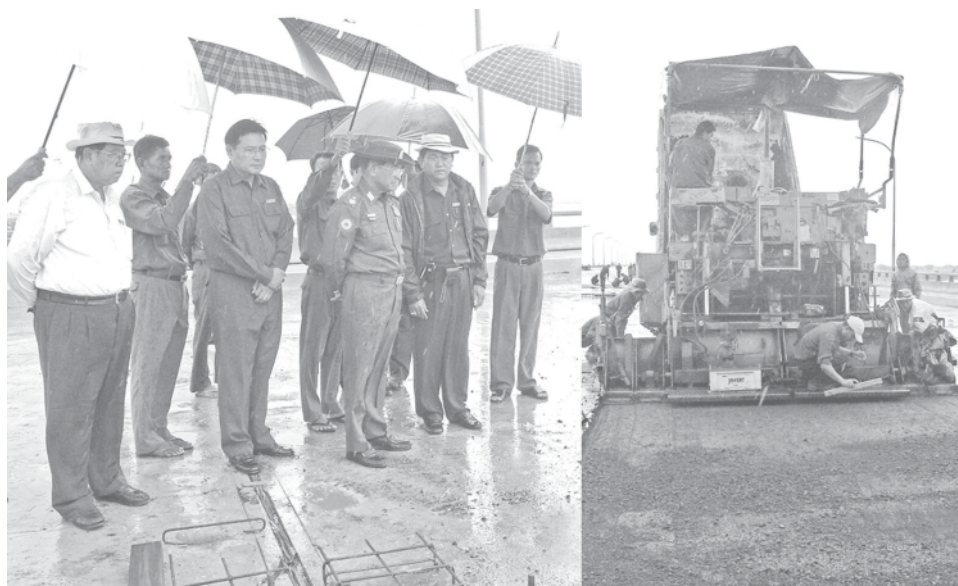
Minister Maj-Gen Saw Tun inspects construction of Dagon Bridge in Seikkan Township. — MNA
