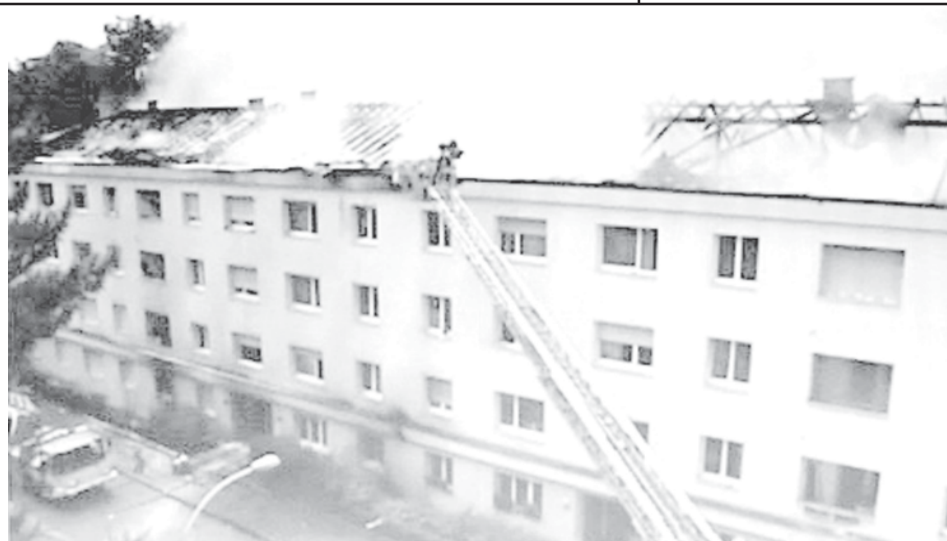
Photo grabbed from local television shows a building burns after it was crashed by an aircraft in Basel, Switzerland, on 23 July, 2007. A small aircraft crashed on Monday into a building in the Swiss city of Basel, killing the pilot and injuring three others, local police said. —XINHUA
