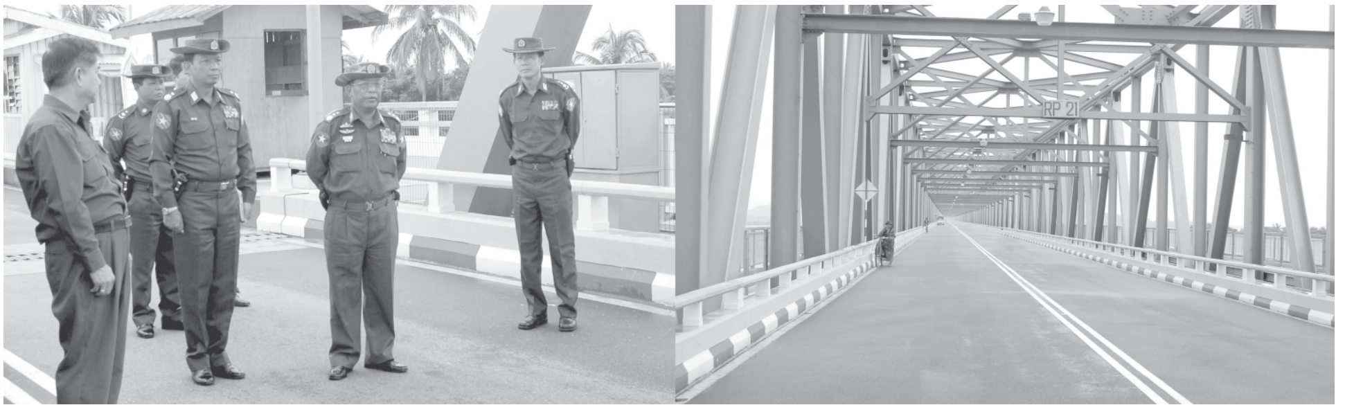
Lt-Gen Maung Bo of Ministry of Defence inspects Thanlwin Bridge (Mawlamyine). — MNA
