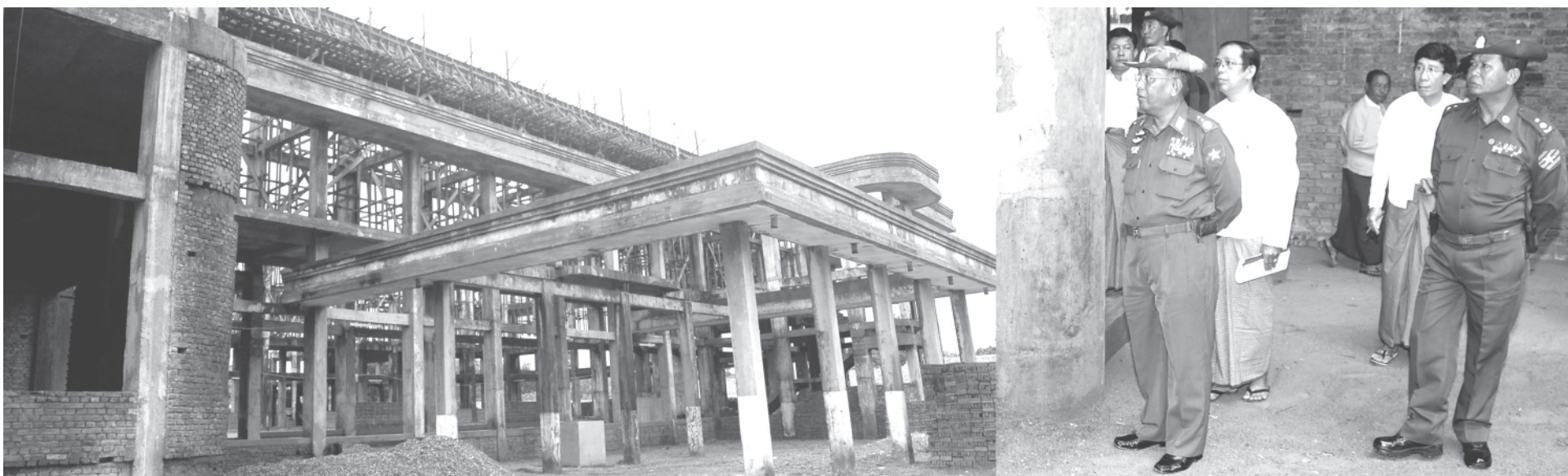
Lt-Gen Maung Bo inspects all-round renovation tasks of Mawlamyine University in Mawlamyine. —MNA
