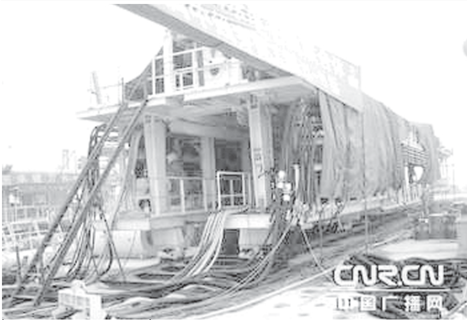
Photo taken on 7 July, 2007 shows the south-to-north water diversion project. INTERNET
