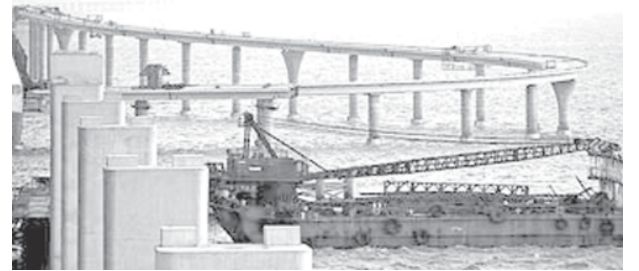
Hangzhou Bay Bridge
