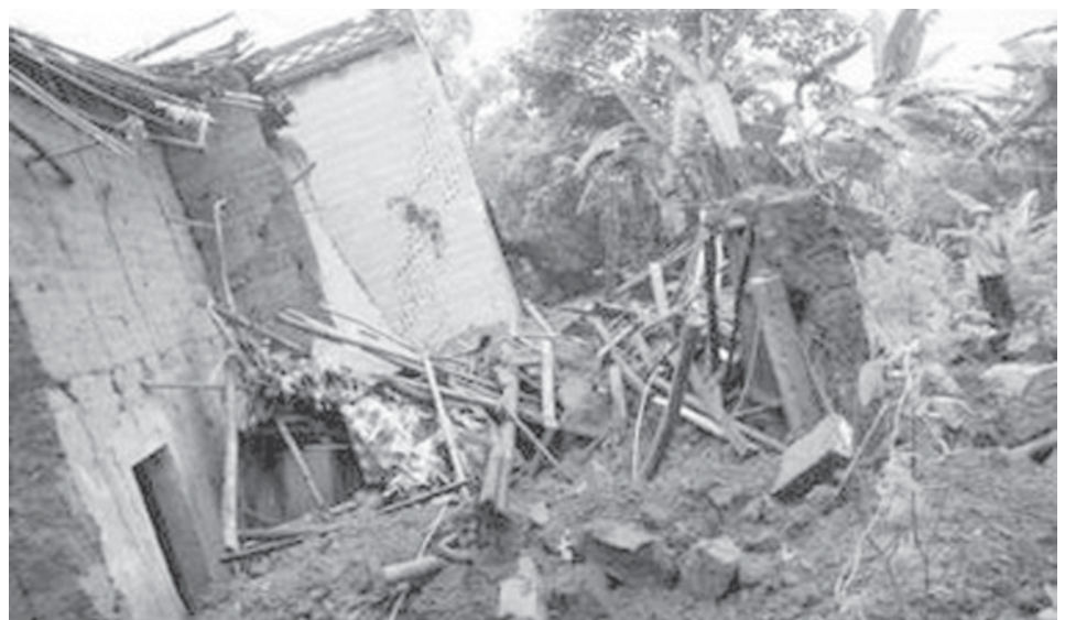
A general view shows damaged houses after a mudslide hit Yunyang county, southwest China’s Chongqing municipality on 22 June, 2007. No casualties were reported, according to local media. — INTERNET
