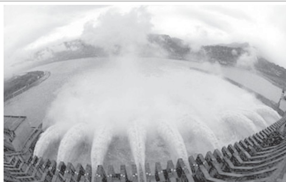
Flood water is discharged through the sluice on the Three Gorges Dam on 19 June, 2007. Continuous downpour on the upper reaches of the Yangtze River has resulted in this year's heaviest flood, with 3,3000 cubic meters of water flowing into the Three Gorges Reservoir every second. The 2007 plan for flood prevention and control has been implemented.—INTERNET
