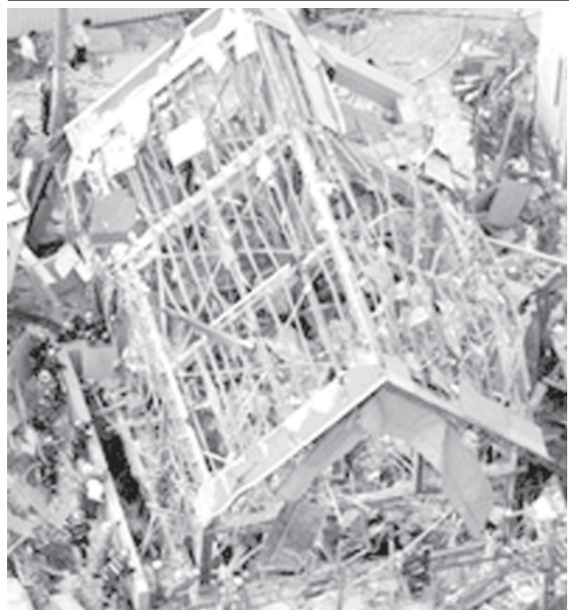
An aerial view shows rescue workers investigate at an annex to a spa’s main building where it exploded in Tokyo on 19 June, 2007. An explosion ripped through a women’s-only hot spring spa in downtown Tokyo on Tuesday, killing at least one woman and injuring at least four other people, police said. —XINHUA
