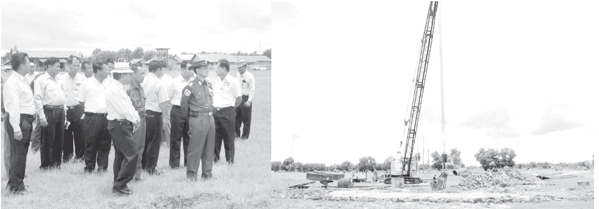
Minister Maj-Gen Khin Maung Myint inspects installation of power line across Bago River.— MNA
