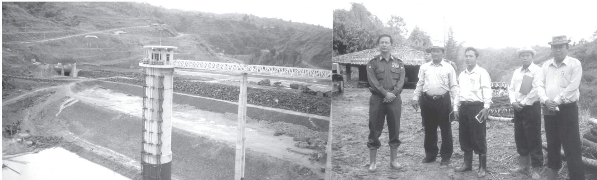
Minister Col Zaw Min inspects Kunchaung Hydropower Project. —MNA
