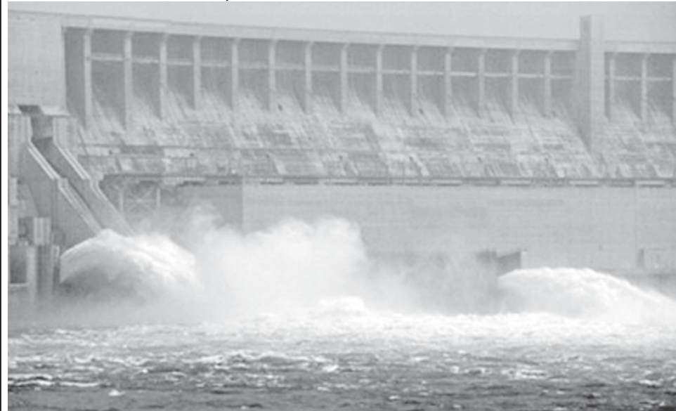
Water gates of the Three Gorges dam in Yichang, Central China’s Hubei Province, open to flush away silt and sand on the riverbed on 13 June, 2007, prior to the rain season. —INTERNET
