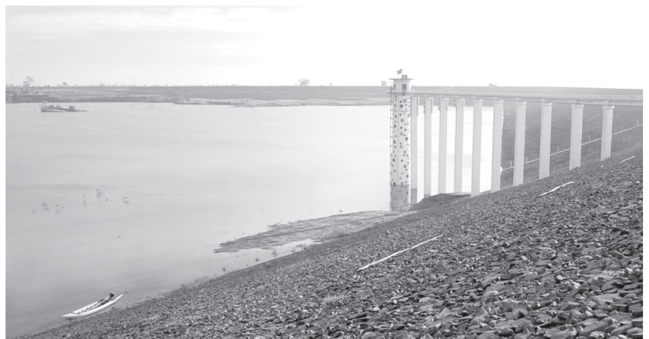
Ma Mya Dam in Myanaung Township, Ayeyawady Division. — MNA
