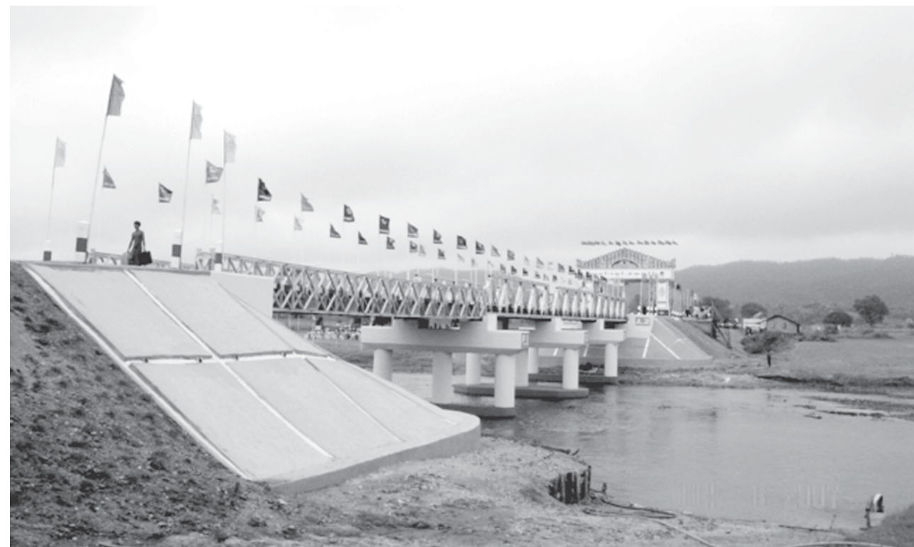
Newly opened Salin Bridge in Salin Township, Magway Division. — MNA
