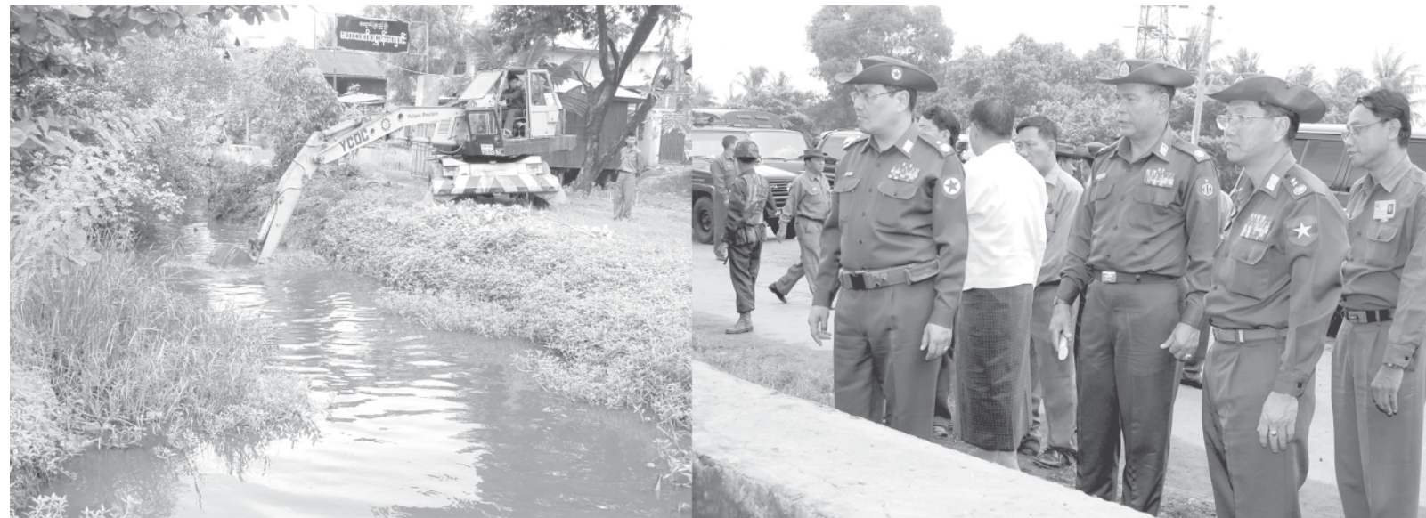
Lt-Gen Myint Swe views dredging of drain in Thakayta Township.—MNA
