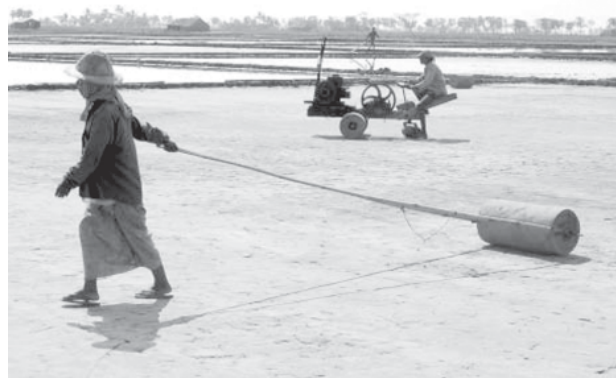
A worker levelling the ground with the use of a roller.
