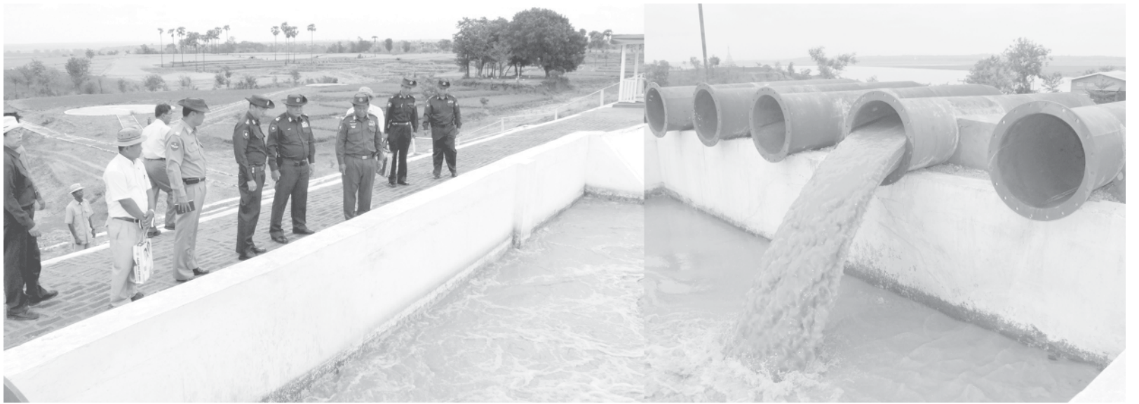
Lt-Gen Ye Myint of Ministry of Defence inspects Thaphanseik River Water Pumping Project. — MNA
