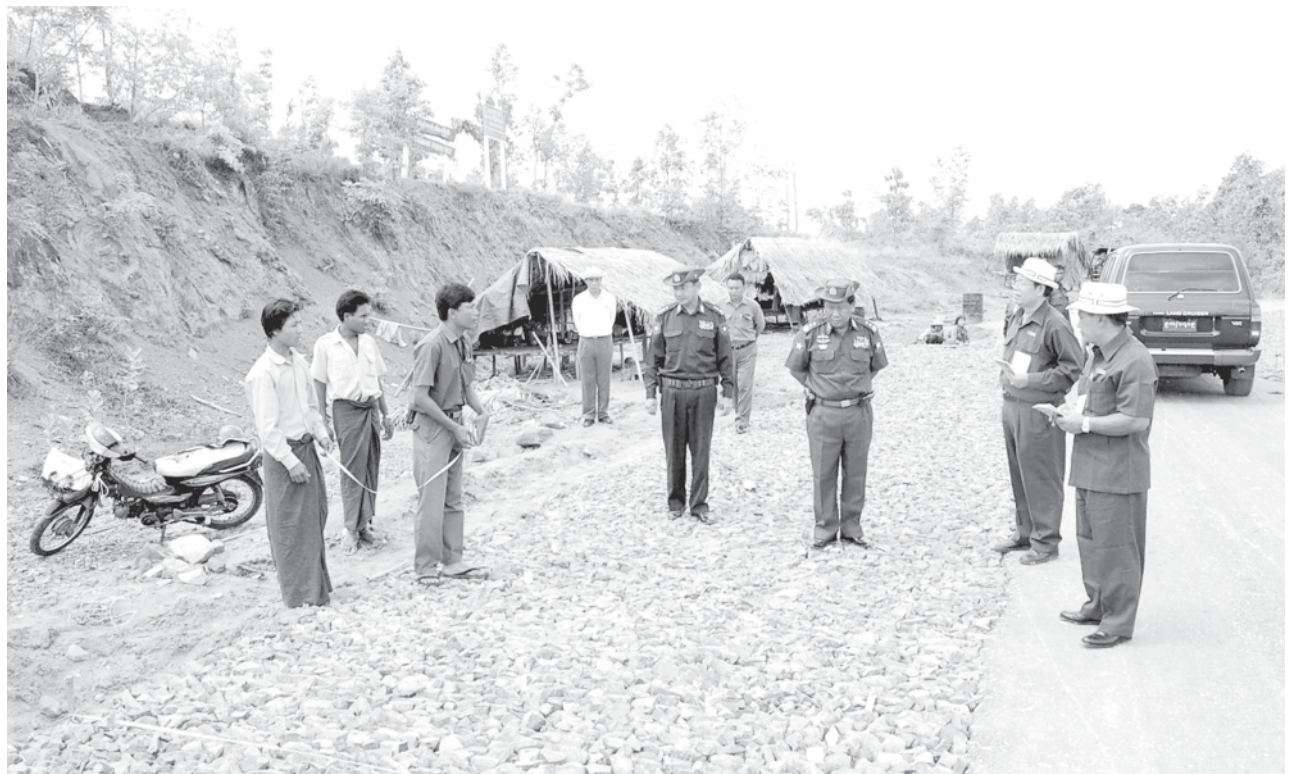
Lt-Gen Ye Myint of Ministry of Defence inspects upgrading of Taungdwingyi road section of Pyinmana-Taungnyo-Taungdwingyi road.— MNA
