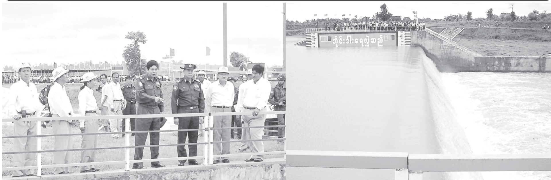
Commander of Southern Command Maj-Gen Ko Ko and Minister Maj-Gen Htay Oo visit Baingda Diversion Dam in DaikU Township.— A & I
