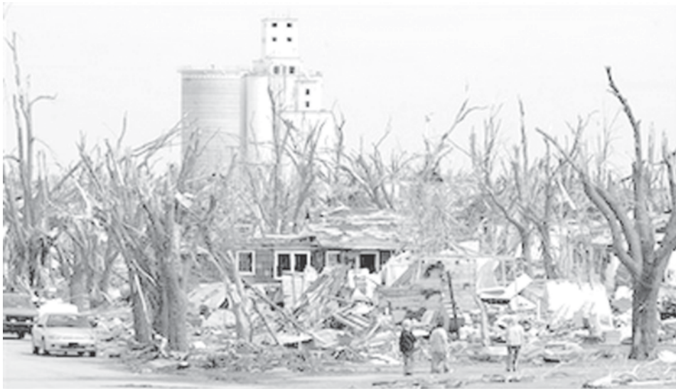
Residents view the damage from Friday's tornado in Greensburg, Kan as they return to town on Monday, 7 May, 2007. The massive tornado, an F-5 category with winds estimated at 205 mph, was part of a weekend of violent storms across the Plains that killed at least 12 people, 10 of them in Greensburg. — INTERNET
