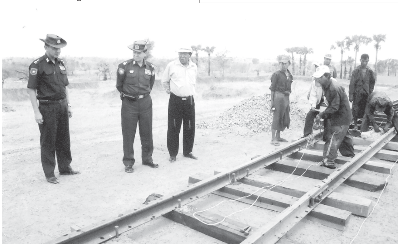
Minister Maj-Gen Aung Min inspects laying railroads on Kyeeni-Chauk Railroad. — MNA
