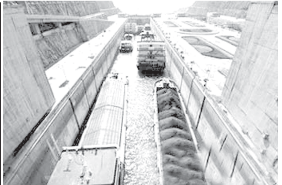
Cargo ships wait to pass a ship lock during trial navigation at the Three Gorges Dam in central China's Hubei Province on 30 April, 2007. The dual-track ship lock of the Three Gorges Dam will fully reopen to traffic on 1 May after more than seven months' construction and trial operations. —XINHUA
