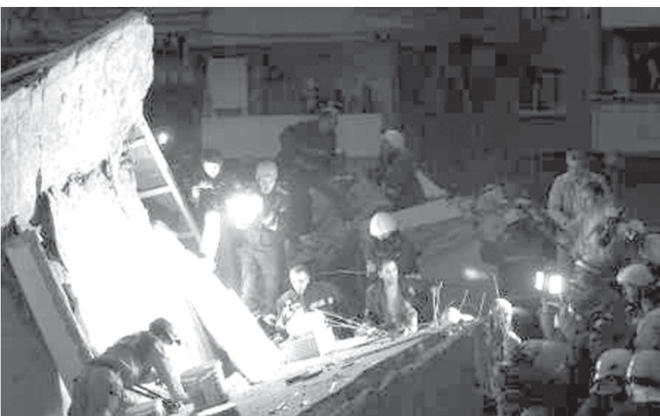
Rescue workers stand on the wreckage of a collapsed eight-story apartment building in Istanbul on 26 April, 2007. The building collapsed in Istanbul on Thursday, but authorities said they did not expect a great number of casualties as people ran away when they heard the building start to crack. — Internet
