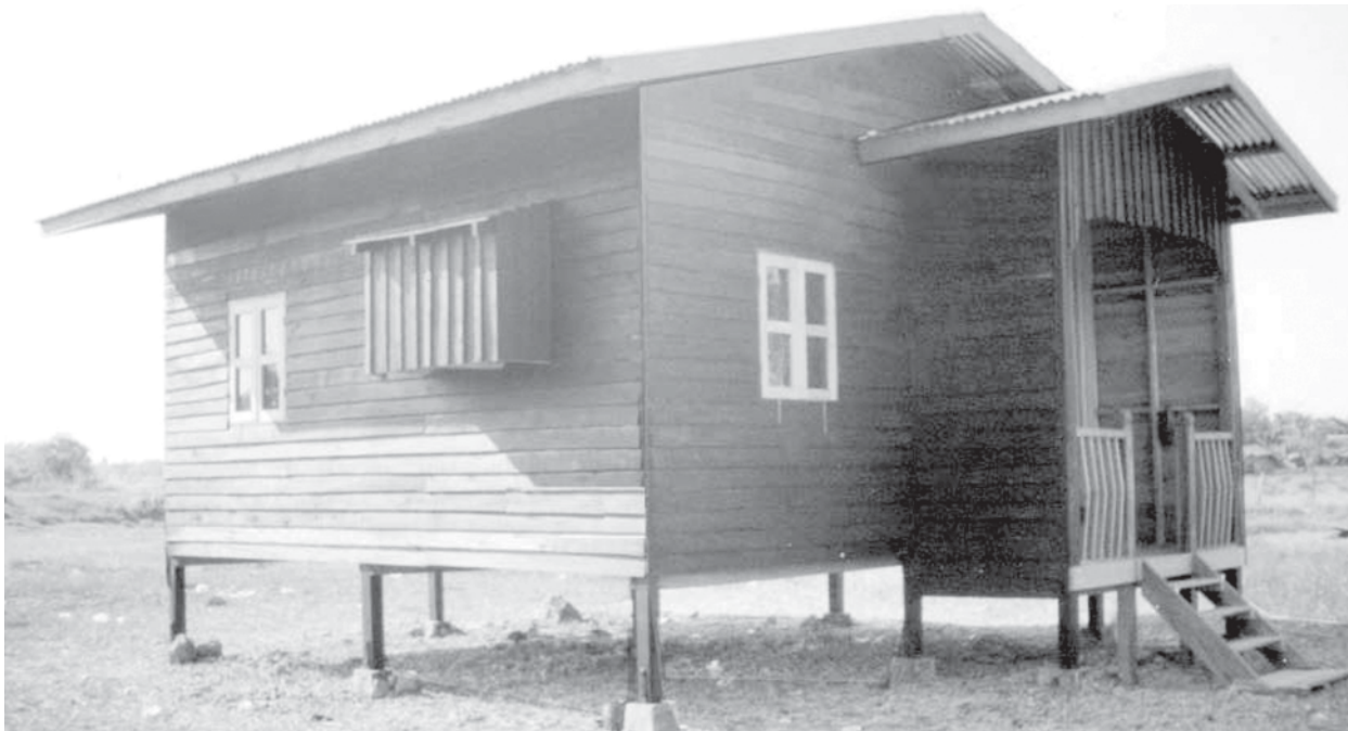
A sample house built with lesser-used species on display at the timber sales centre in Dagon Myothit (North), Yangon Division.
