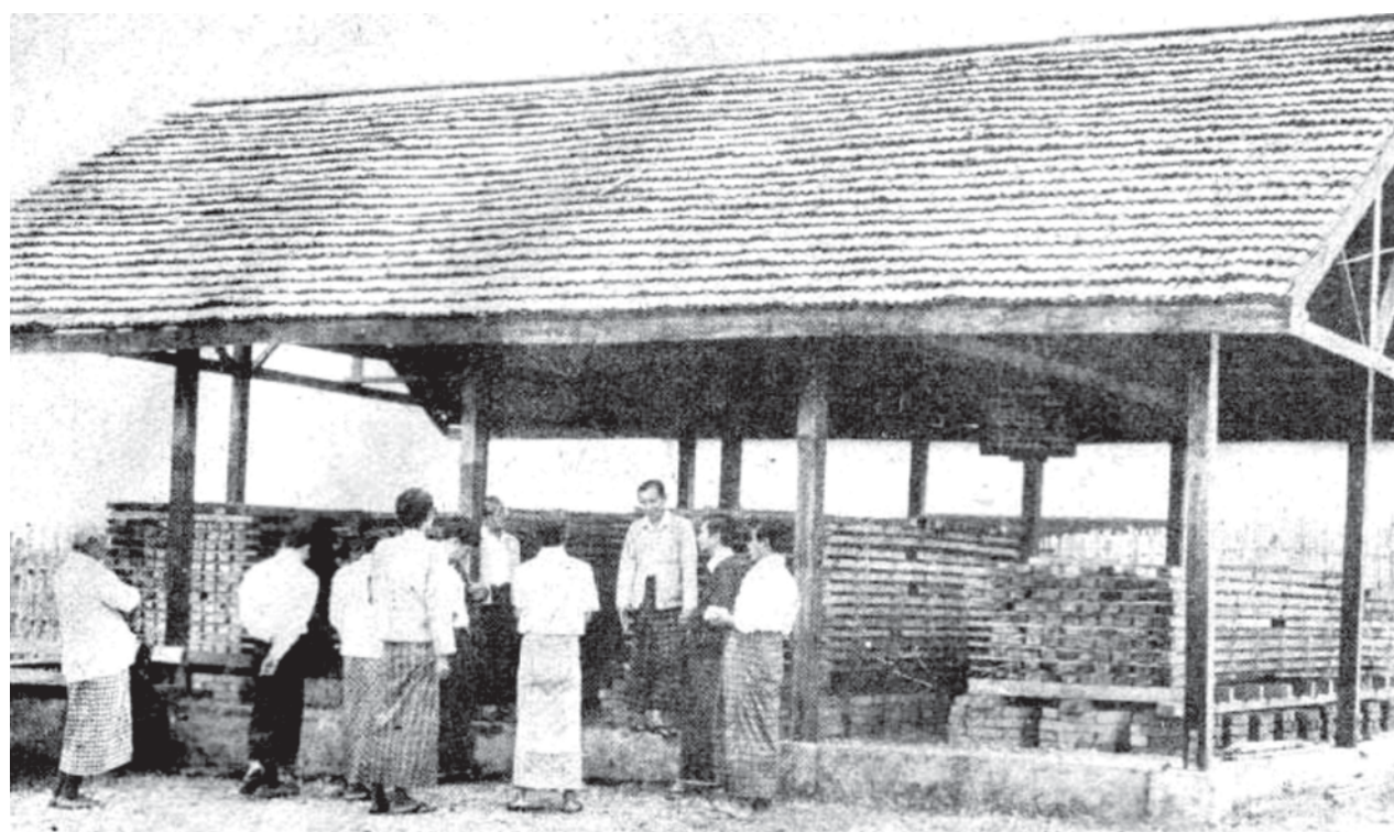
Bamboo shingles used in roofing a hut of research unit of Yezin University in January 1979 are still good at present.
