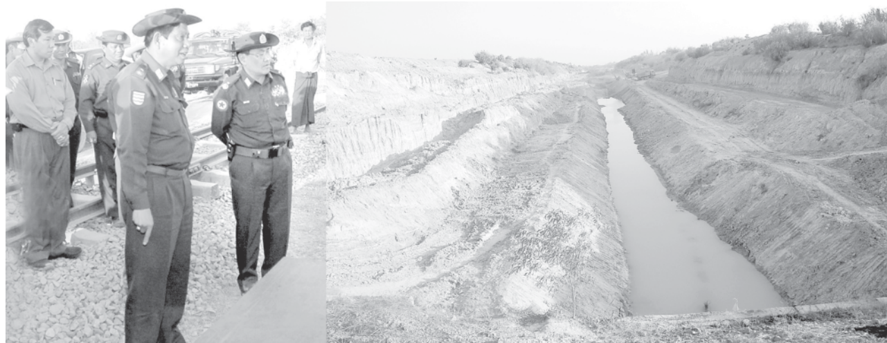
Commander Maj-Gen Hla Htay Win and Minister Maj-Gen Htay Oo inspect condition of main canal of Lagunpyin Dam in Hlegu Township. — MNA
