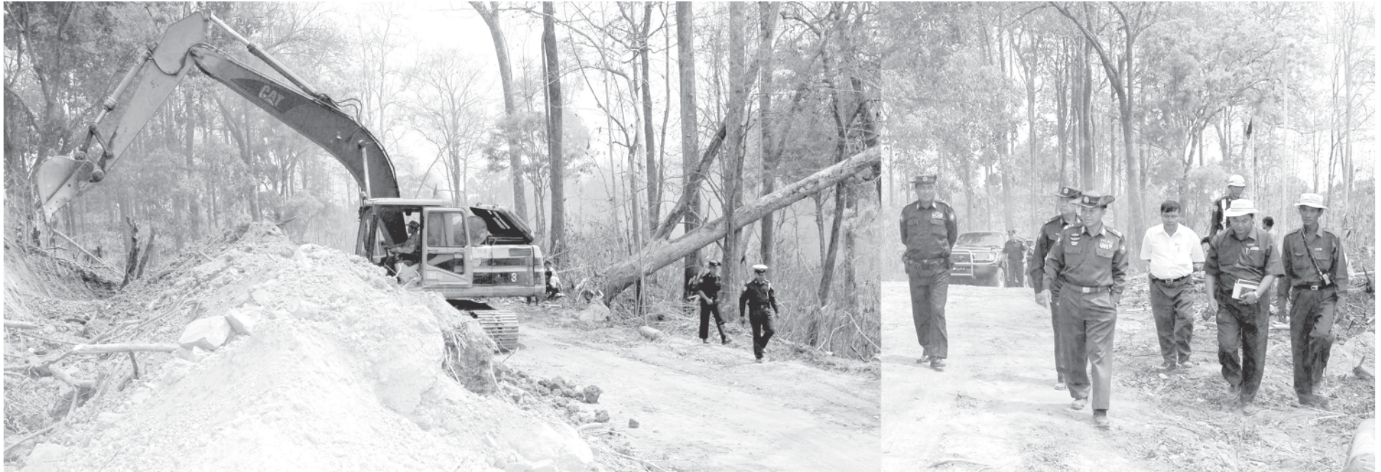
Lt-Gen Khin Maung Than inspects the upgrading of Pyay-Paukkhaung-Toungoo Road. — MNA
