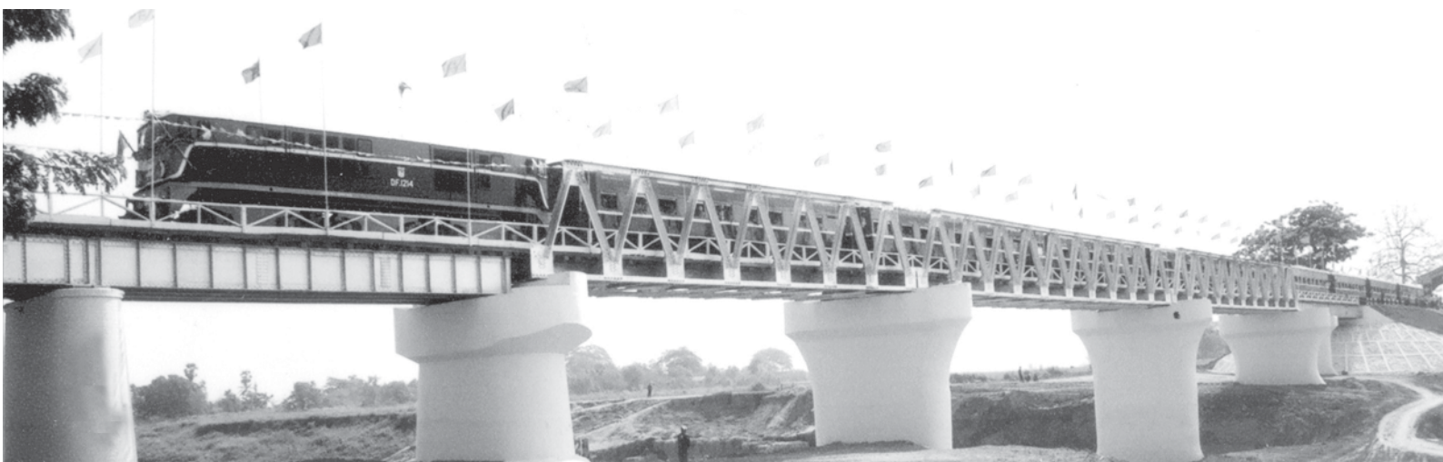
Newly opened Phatashin Bridge.—MNA
