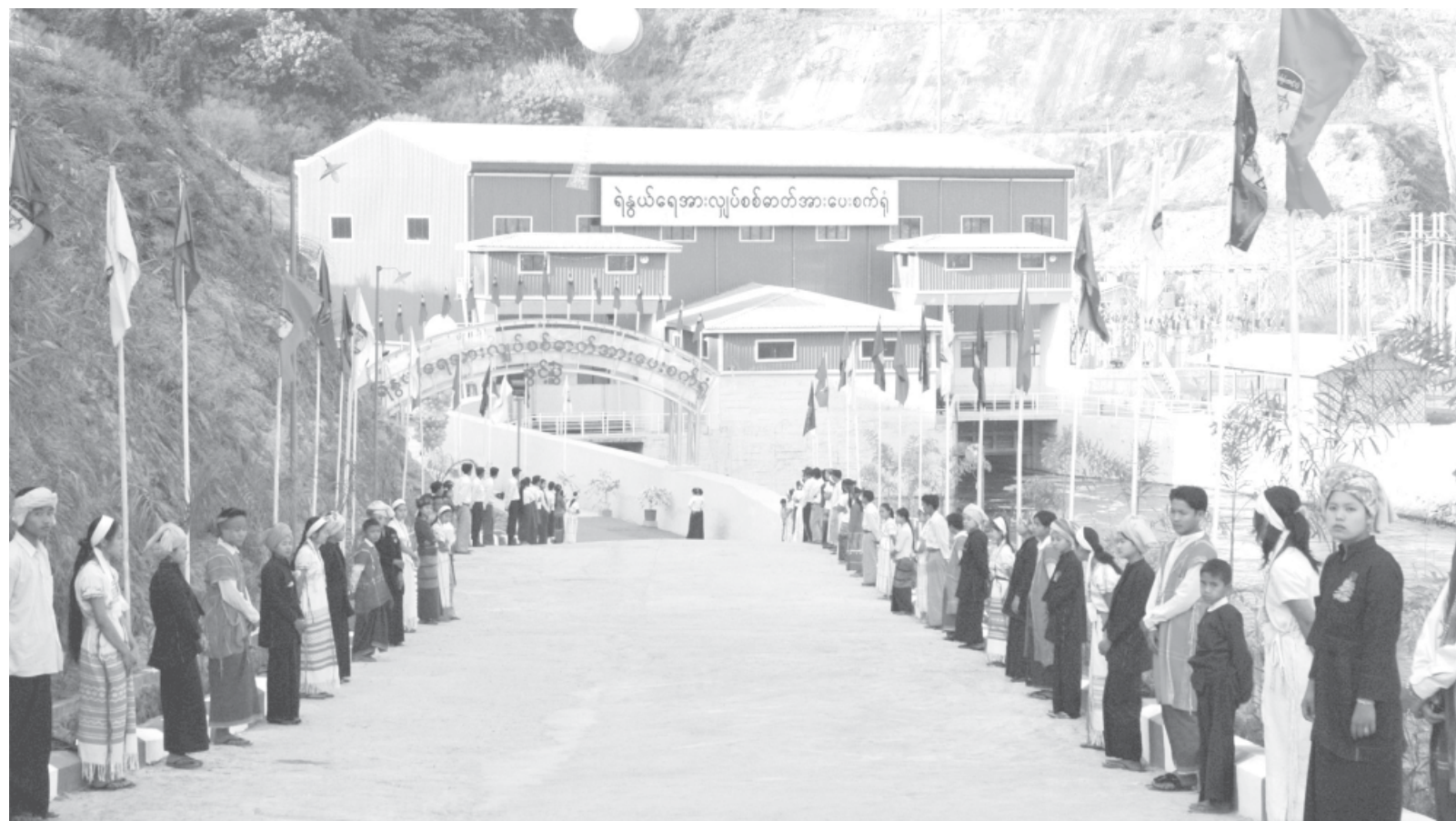
Yenwe Hydel Power Plant near Myochaung Village in Kyaukdaga Township can generate 123 million kilowatt hours annually.
