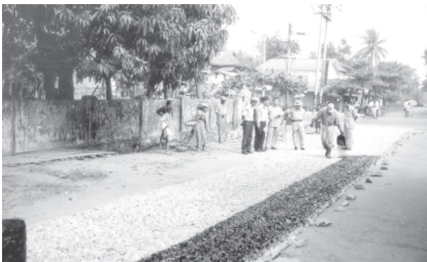
Director-General U Myo Myint inspects road repairs in Bago. — H
