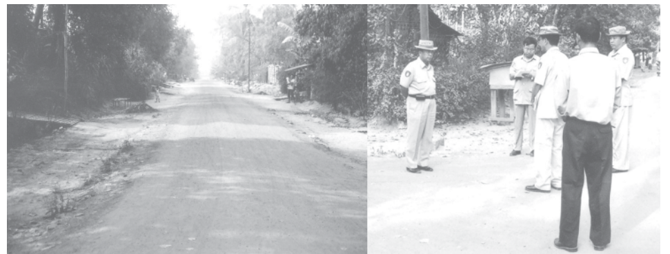
U Myo Myint of DAD inspects Maggin road constructed by Thanlyin Township DAC. — DAD
