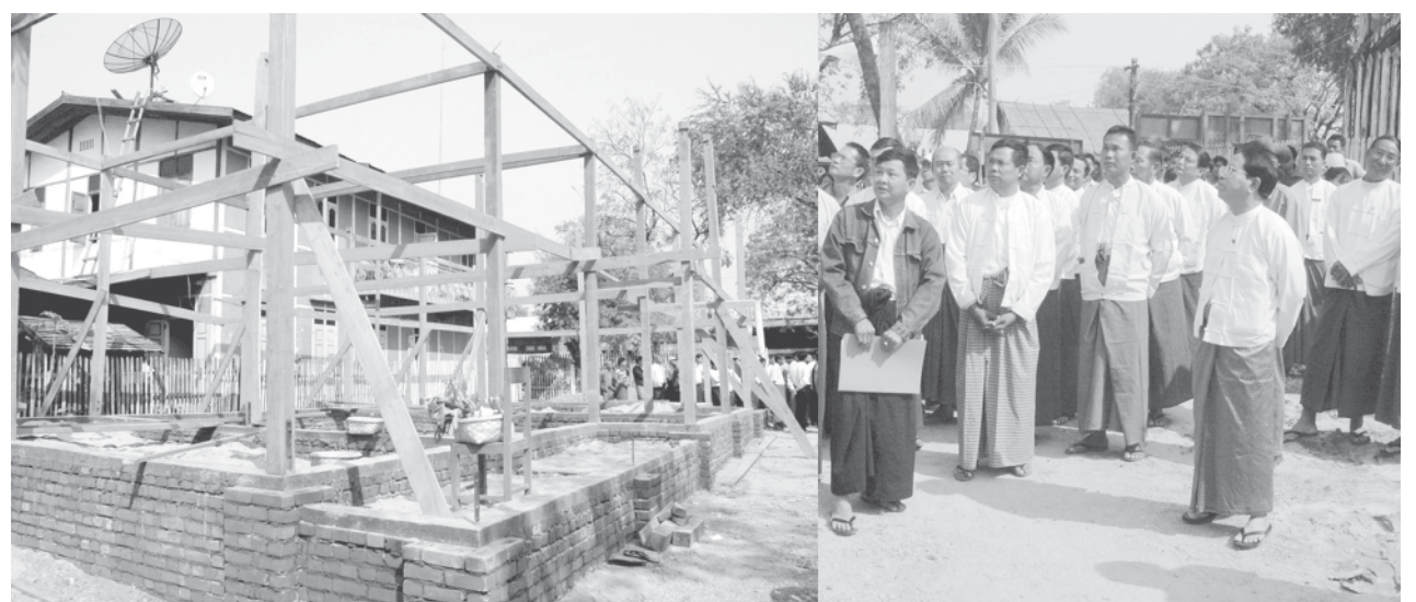
Minister for Information Brig-Gen Kyaw Hsan inspects construction of rural health care centre at Mintaingbin Model Village.— MNA
