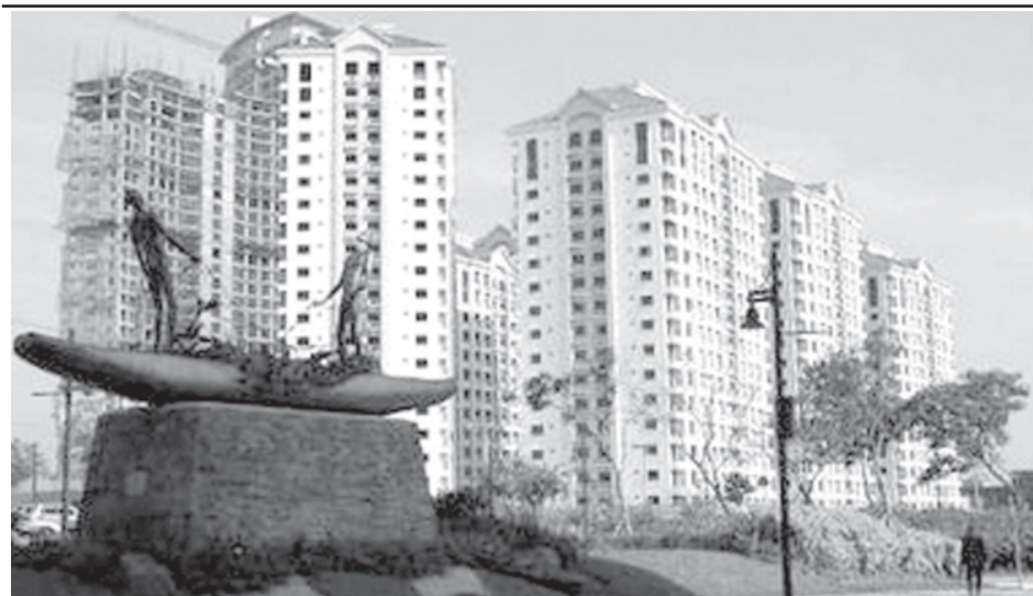
A woman walks past newly constructed condominium buildings in Manila's financial district of Makati on 12 March, 2007. Across the Philippines' sprawling capital city, the small ranks of the wealthy are increasing as record remittances from nearly 9 million Filipinos — driven abroad by poverty and a lack of opportunity — fuel consumer demand and a property boom. — INTERNET
