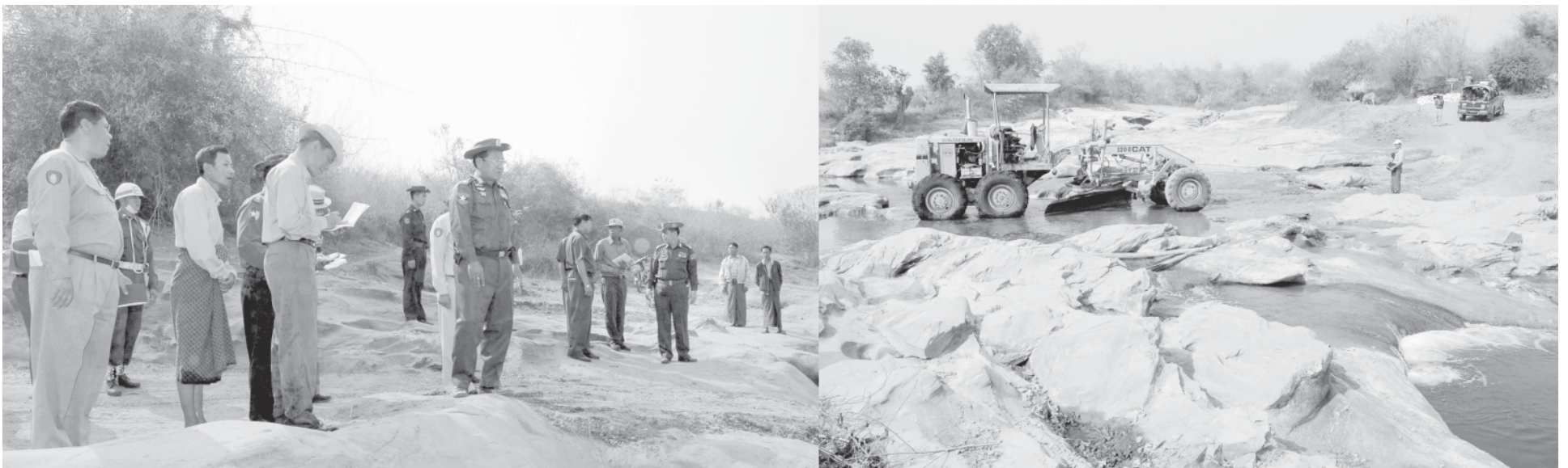
Lt-Gen Ye Myint inspects a site chosen for building an embankment on Kotkoai Creek. — MNA
