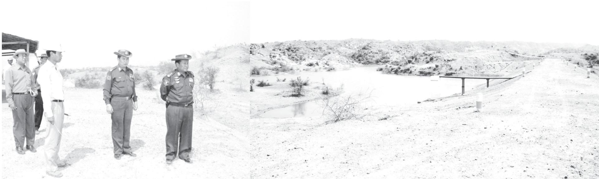
Lt-Gen Ye Myint of Ministry of Defence inspects construction of Zawkanar Creek Dam — MNA
