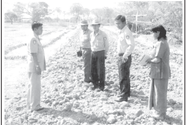
RURAL ROAD INSPECTED: Director U Tin Hlaing of Development Affairs Department (Head Office) inspected progress of Kannyiko-Taungpohthaya rural earth road being constructed by Zigon Township DAC for 2006-07 financial year recently. Township DAC Executive Officer U Tin Aung Saw and Junior Engineer-2 Daw Saw Swe Win reporting on construction of the road.
