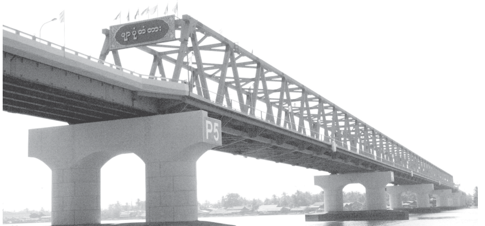
Progress of Pyapon Bridge linking Pyapon River between Ward 1 in Pyapon and Ohnbin Village in Dedaye Township. — MNA
