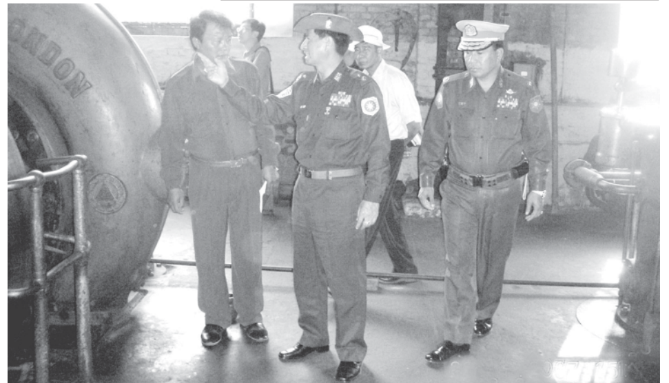
Commander Brig-Gen Aung Than Htut and Minister Maj-Gen Khin Maung Myint inspect Mansanyaykya Hydel Power Station in Lashio. — MNA
