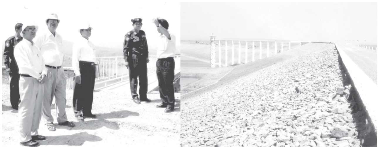
Minister for Agriculture and Irrigation Maj-Gen Htay Oo visits Ma Mya Dam Project.— A&I
