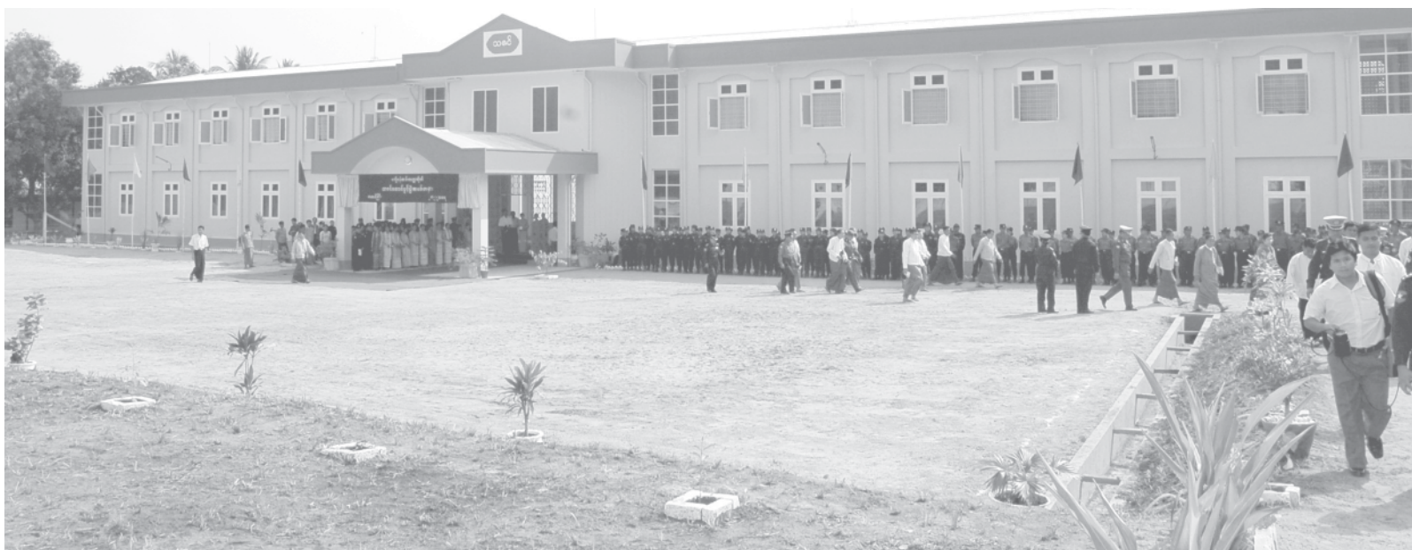
Two-storey Thazin Hostel for women's company in Central Institute of Civil Service. — MNA
