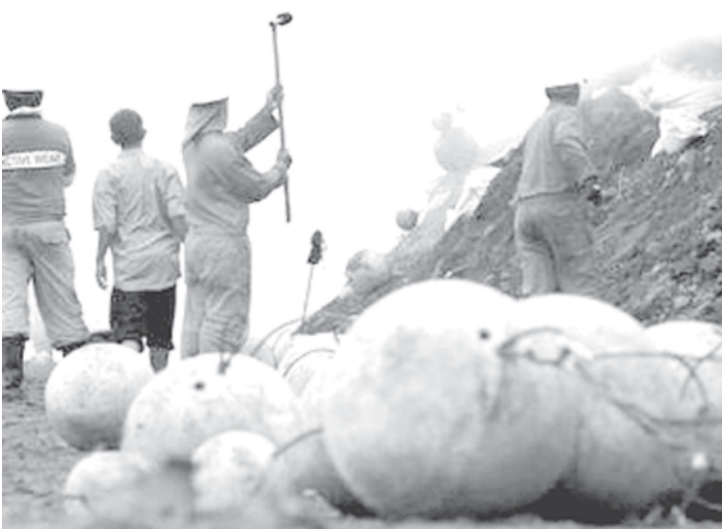
Indonesian engineers drop concrete balls into a mud volcano in Sidoarjo, East Java province on 26 Feb, 2006. The balls were used to reduce the torrent of sludge that has displaced about 15,000 people, a scientist said. INTERNET
