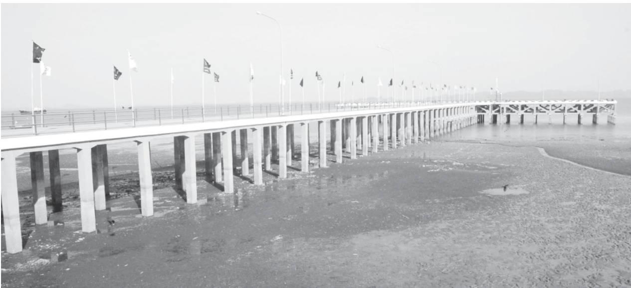
Newly opened Phaungdawgyi Concrete Jetty at Sittway Port.— MNA
