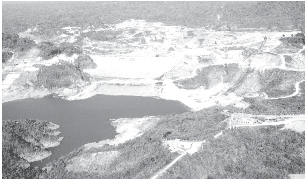
Khabaung Dam Project. — MNA
