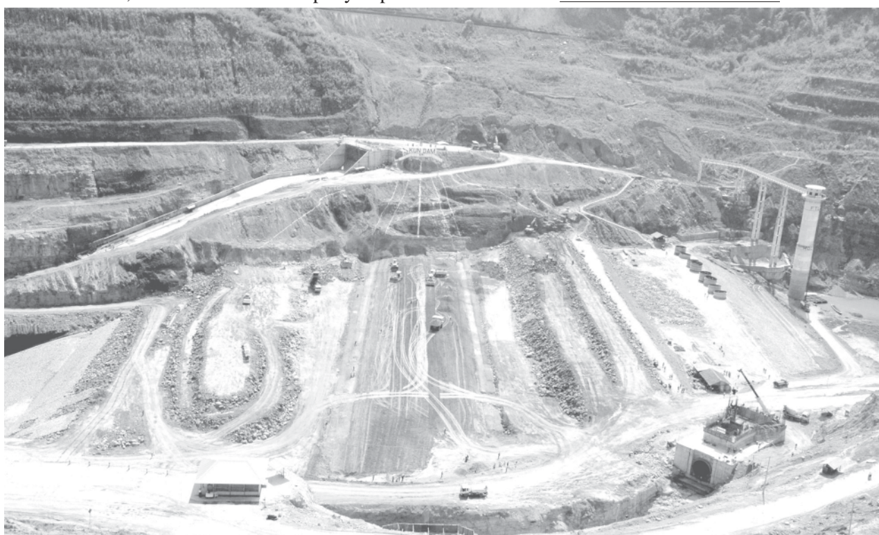
Kunchaung Hydel Power Project. — MNA
