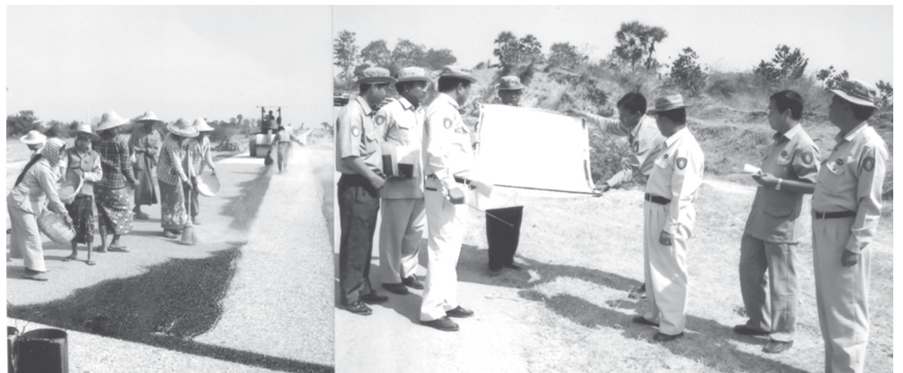
Officials of Development Affairs Department inspect district-to-district road between Mandalay and Magway.
