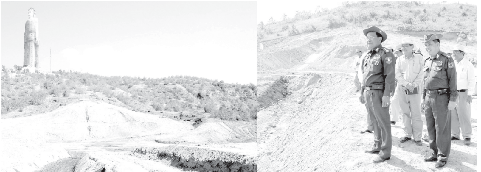
Lt-Gen Ye Myint inspects construction of Bawditahtaung Dam.—MNA
